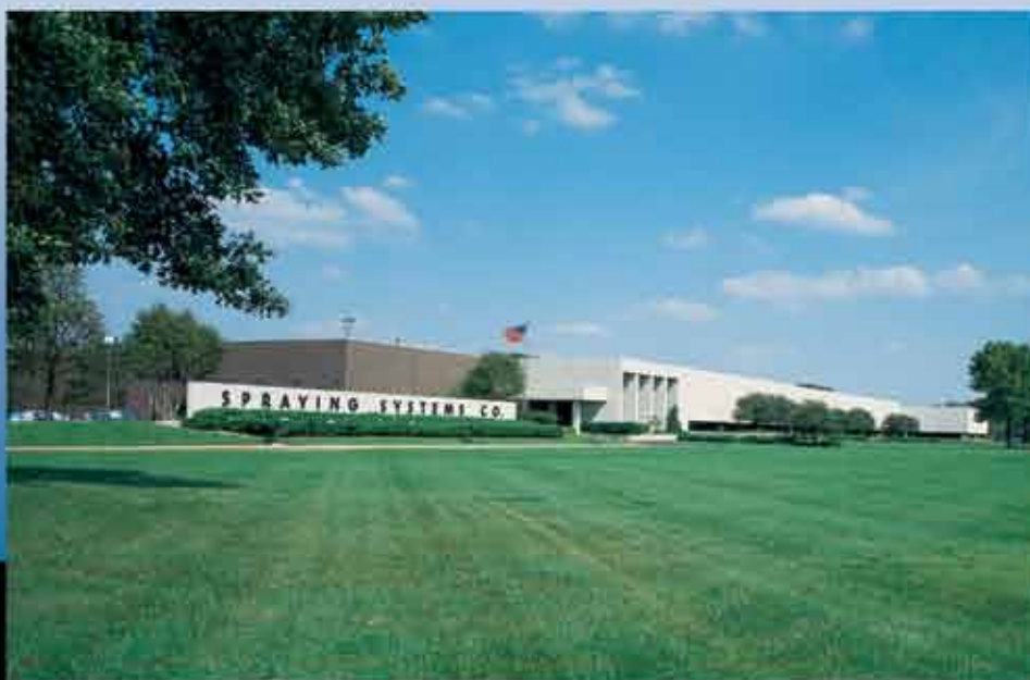
Spraying Systems Co. World Headquarters Wheaton, Illinois USA
